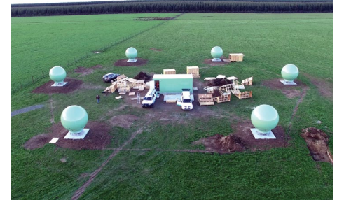
MEOSAR satellite receiving station under construction
